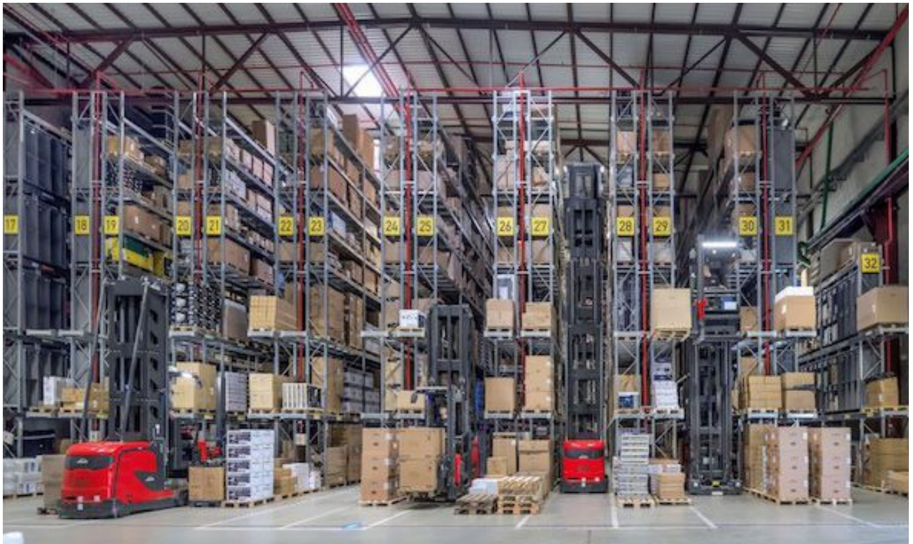
Linde has provided autonomous lift trucks for very narrow aisles at Wagner eCommerce. Source: Linde Material Handling
